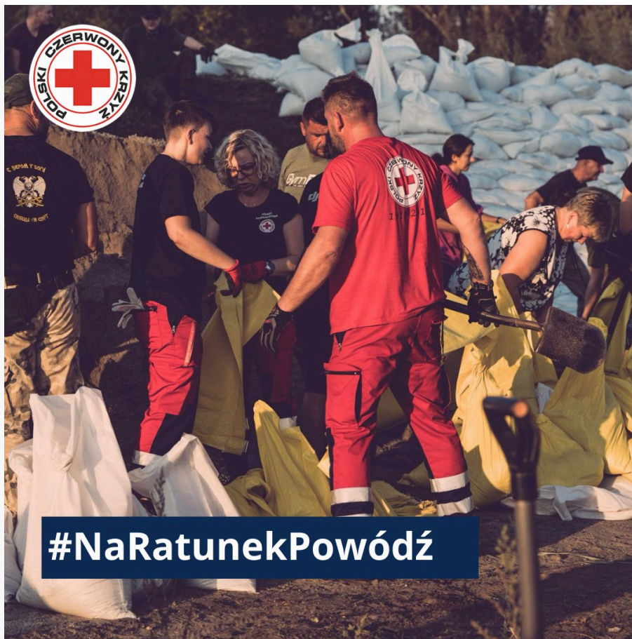
Dike strengthening, September 2024. Source: PRC
